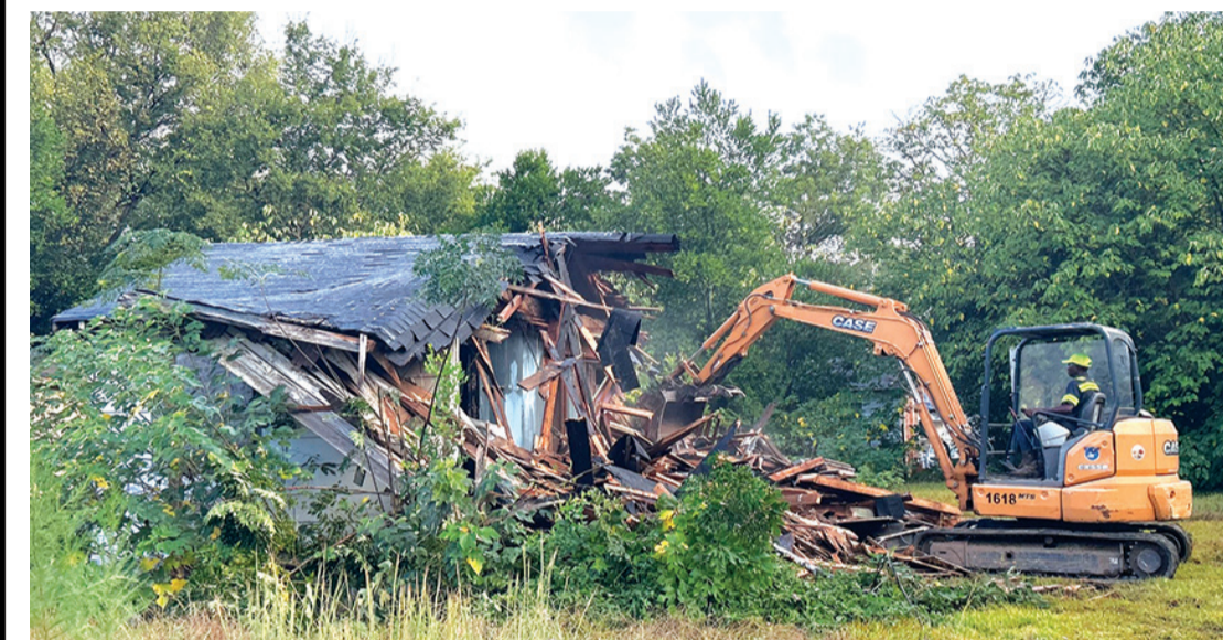
230 Cliett Street before demolition.
