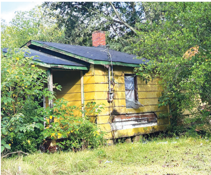
524 & 526 Cliett Street before demolition.
